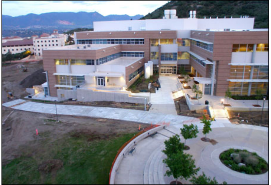
The UCCS Science and Engineering Building will use thin-film solar panels for energy.
